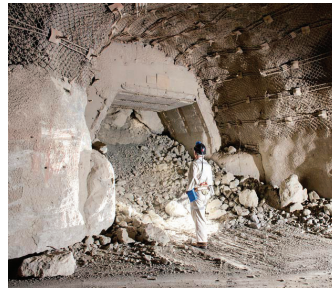
Underground at the Finsch mine in South Africa
